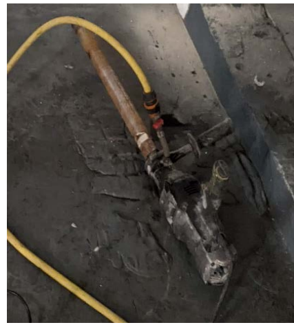
A4.2: Column Coring
