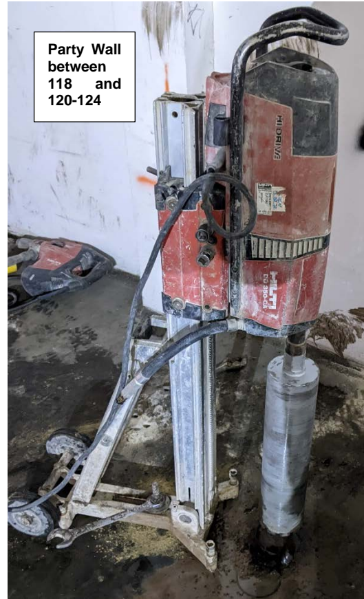
A4.8: Stich (core) Drilling – First Floor
