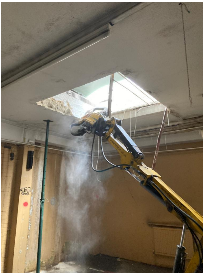
A3.17: Test No. 17 – Munching on Slab, Roof.
