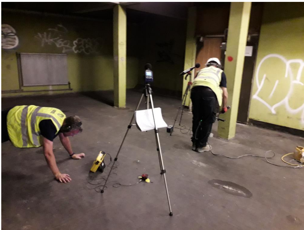
A3.6: Test No. 6 – Boring Holes to Coring Column, Front Room, Basement.
