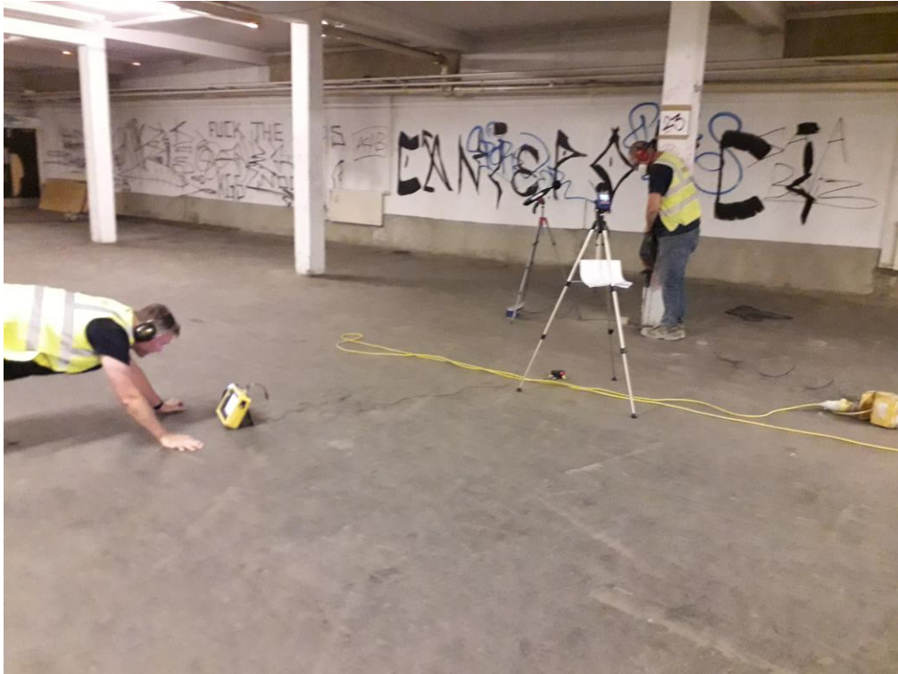
A3.13: Test No. 13 – Percussive Drilling to Slab, Main Room, Basement.
