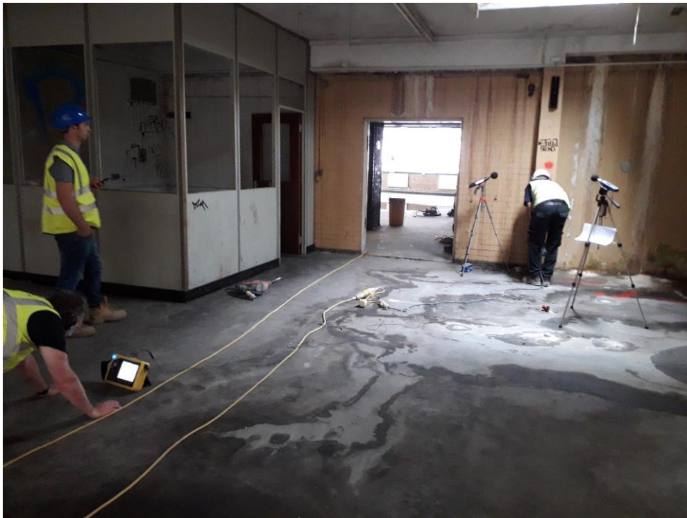
A3.8: Test No. 8 – Boring Holes to Coring Column, Lift Shaft, First Floor.
