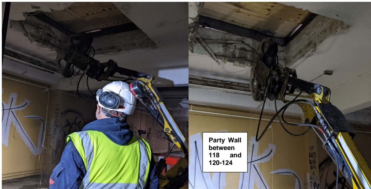
A4.9: Brokk 90 – Slab breaking, First Floor Roof
